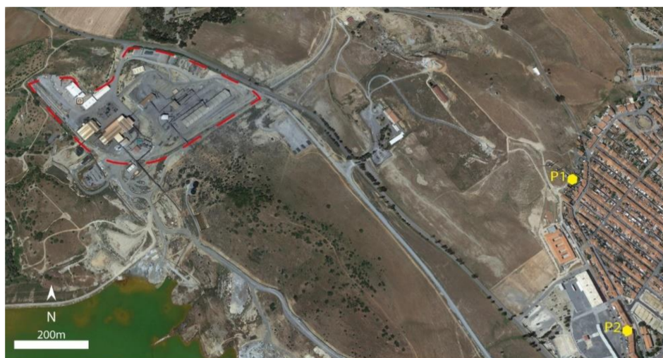
Figure 2. Localization of the ore processing plant of the Aljustrel mine (red line) and the sampling points: P1 and P2 at a distance of 1.2 km and 1.44 km, respectively (source: Google Earth).
