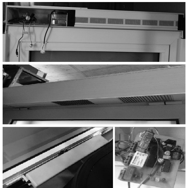
Fig. 2. Prototype of the mechanical ventilation subsystem of the Smart Window hybrid ventilation system: centrifugal blower (top); automatically operable window actuator (lower left) and control board (lower right).
