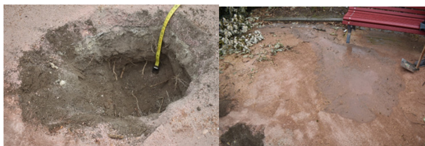
Figure 16. Ground cover and permeability test (August 2022).
