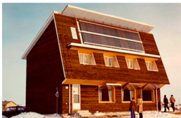
Figure 1. Saskatchewan Energy Conservation house designed by the Illinois U. demonstrated passive technology in 1978 (Regina, SK, Canada). Solar-exposed surfaces with large windows are inclined. Evacuated solar pipes are placed on the attic level. It was provided with an air–air heat pump and polyethylene-based heat recovery ventilator. Courtesy of Harold Orr.
