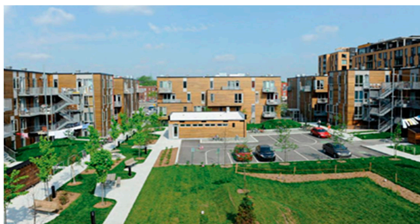
Figure 6. An affordable, low-rise, energy-efficient multi-unit residential building, “Atelier Rosemount”, in Montreal. Note the rain retention basin in the bottom right (credit Nikkol Rot).
