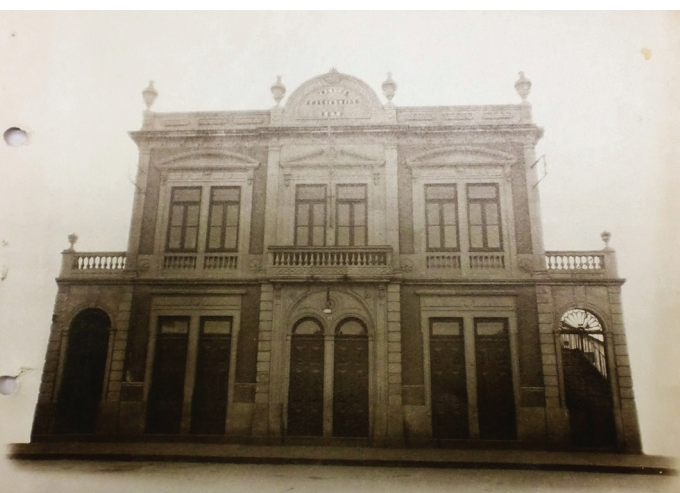
Fig.24 Fachada principal original
