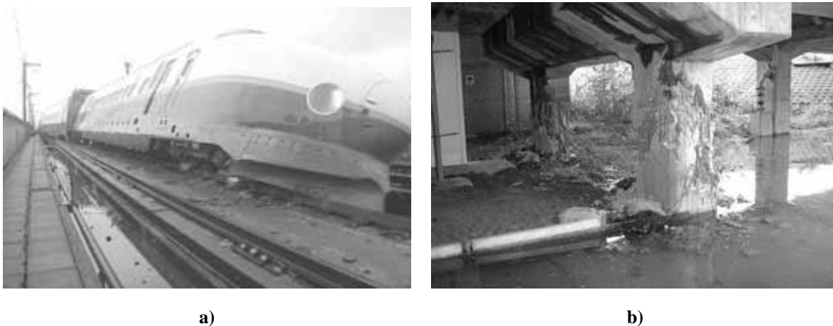
Figure 2-12 Liquefaction damages to the rail infrastructure from the 2004 Niigata Ken Chuetsu earthquake: a) the derailed Shinkansen train and b) damages to the viaduct columns where the derailment occurred. (Ogura 2006).
