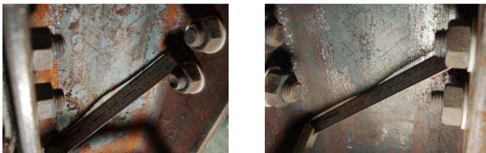
Figure B.15: Local deformation of the column web on the bottom part (level of the bolt rows 3 and 4) under hogging bending moment (test 3 – 700°C and no axial restraint to beam)
