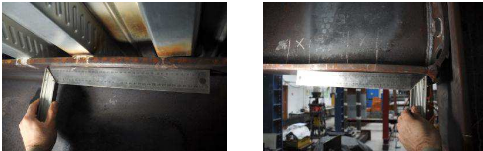
Figure B.20: Local deformation of the flanges from the right beam (view from the back / test 4 – 500°C and total axial restraint)
