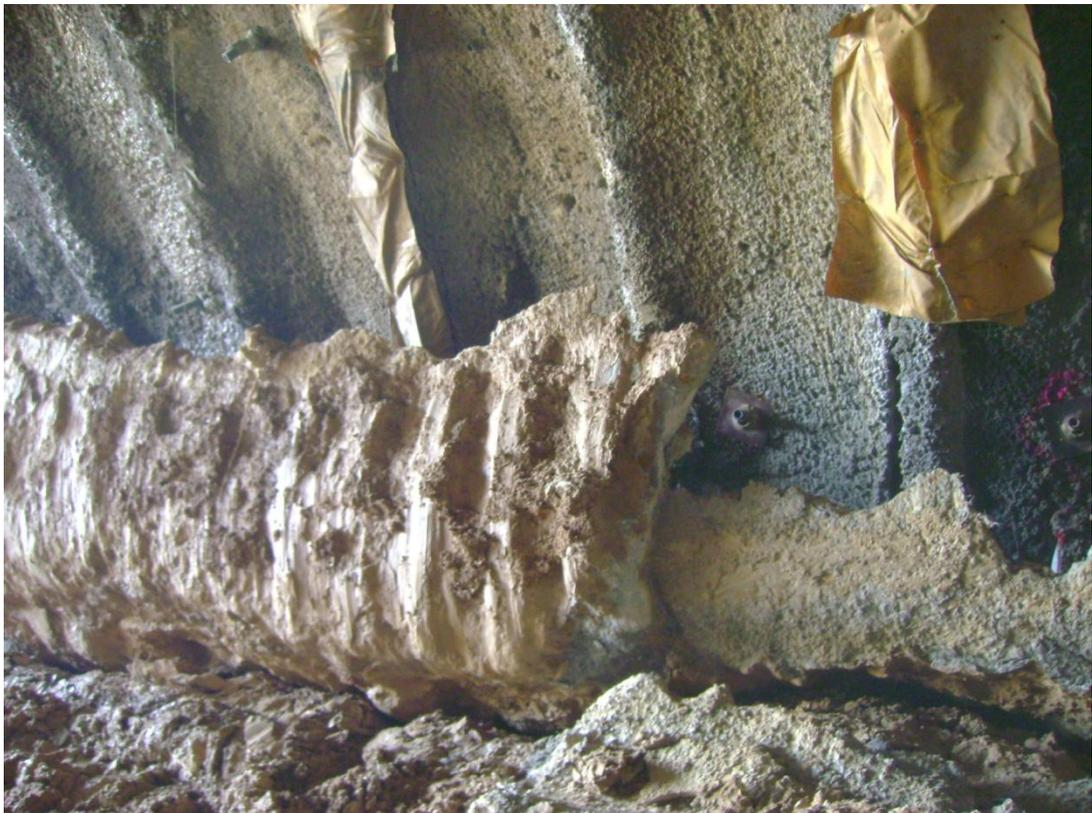
Fig. 8 View of the provisional mortar gutter rotated upwards on the left side of the tunnel
