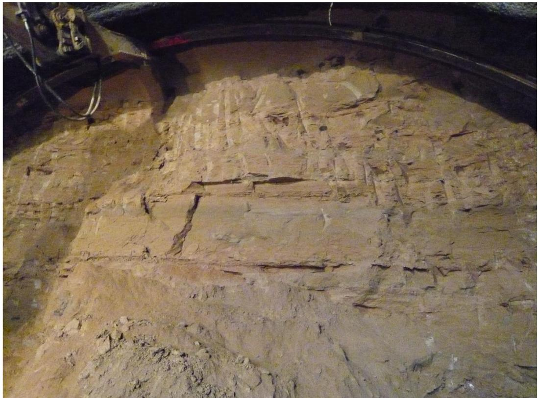
Fig. 4. Excavation front in progress, presenting high homogeneity and good stability
