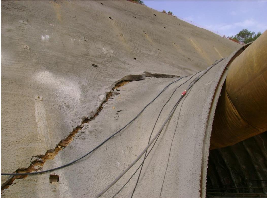
Fig. 7. Fissure developed above the North portal lining.
