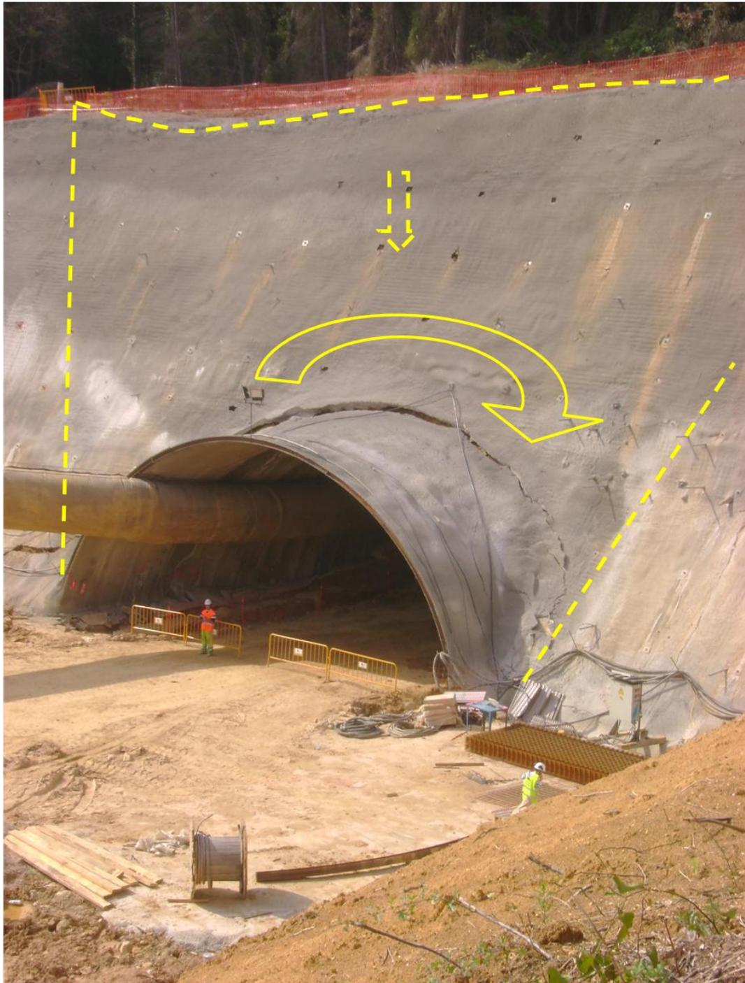
Fig. 6 Overview of the North portal after the collapse. The horizontal dashed line highlights the 0.5 m depression at the top of the portal. The dashed harrow points the downward movement. The vertical and inclined dashed lines indicate the two longitudinal fissures 30 m long, The circular arrow indicates the circular shape of the fissure above de tunnel lining
