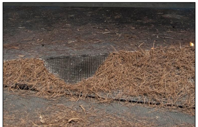
Fig 6-22 a typical shape of burned area on the windward face for inclinations less than 35-deg, the image is from test (3D3)
