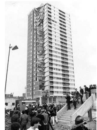
c) 1968, Ronan point, London – accidental gas explosion.
