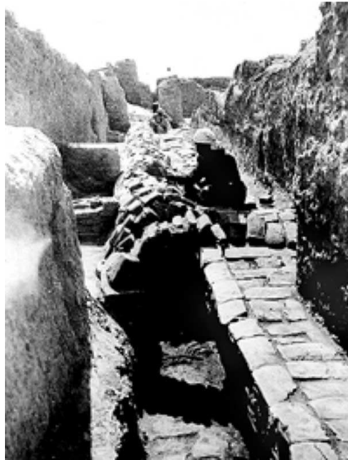
Figure 2.1 – Sewer pipe in the ruins of Ancient Babylon (U.S. National Archives)
