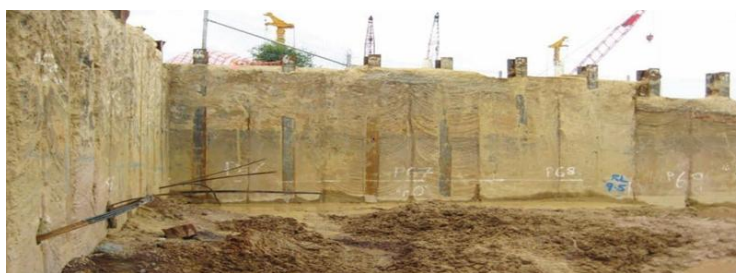
Figura 2.3 - Obra executada com Painéis de Cutter Soil Mixing (Civil Works@, 2015).
