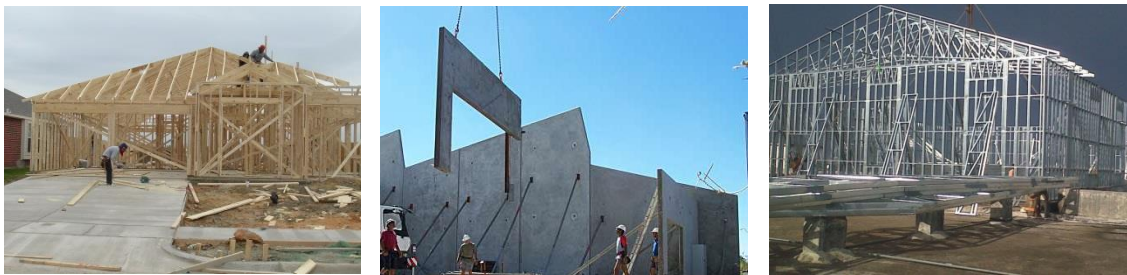
Figure 18 Wooden, concrete and light steel framing prefabricated construction examples
