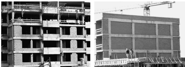
Fig. 1. Typical concrete structure of Portuguese buildings filled with non-loadbearing masonry walls.
