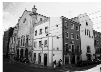
4. The present view of Rua João de Ruão (north side) and Rua da Sofia (east side). Photo: Vítor Murtinho.
