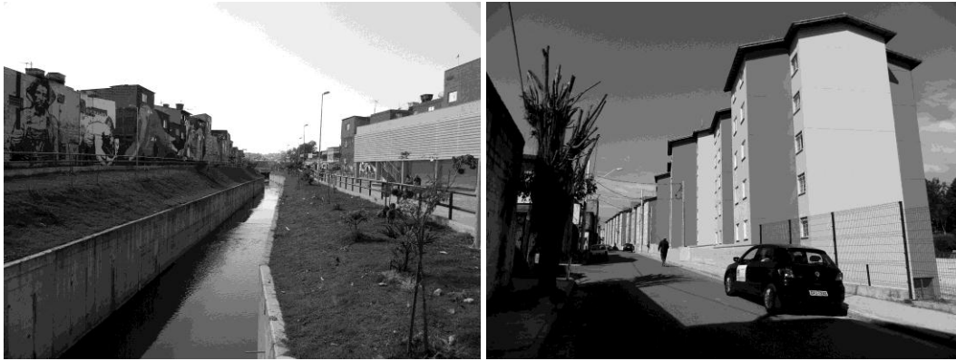
Conventional stream canalization solutions (left) and housing units (right). Source: Luciana Ferrara (2012)
