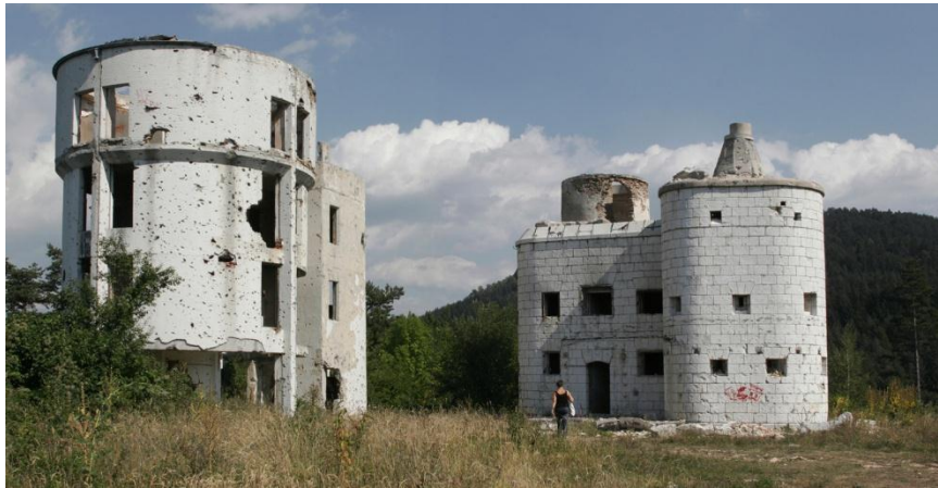
Figure 6. Destroyed observatory buildings. Photograph by Zoran Kanlić, May 2012.
