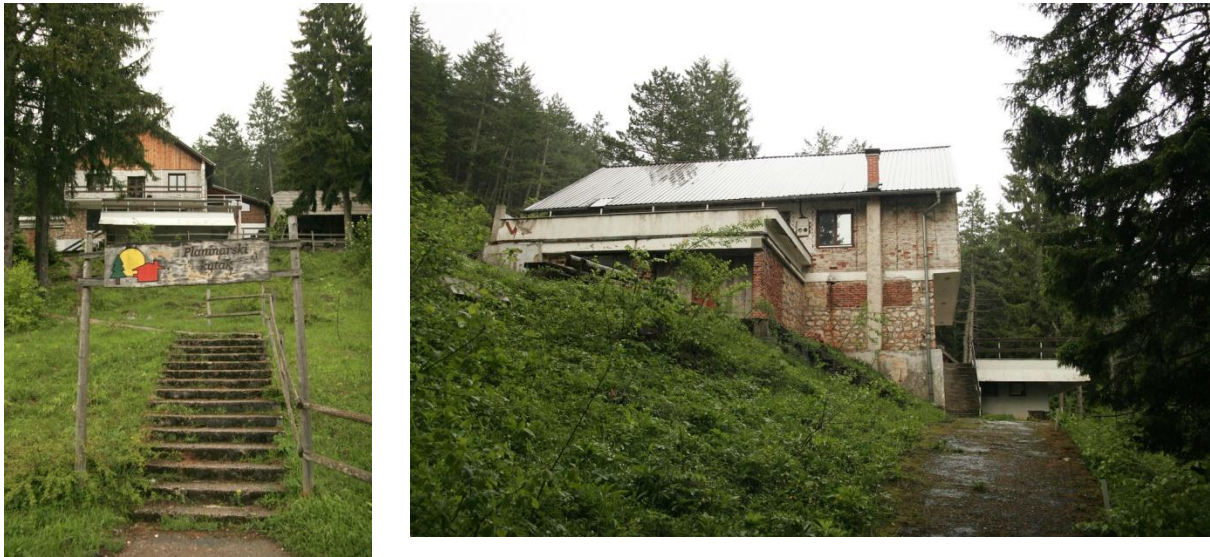
Figure 7. Renovated mountain hut 'Planinarski kutak/Mountain Corner'. Photographs by Zoran Kanlić, May 2012.
