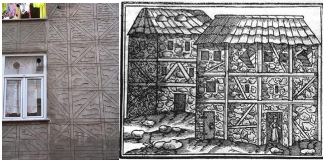
Figure 9. Gazi, the decoration on the façade of an apartkondu (left) and two buildings erected with the technique hıms in a xylography of the seventeenth century (right). Note: Image on right is copyright free.
