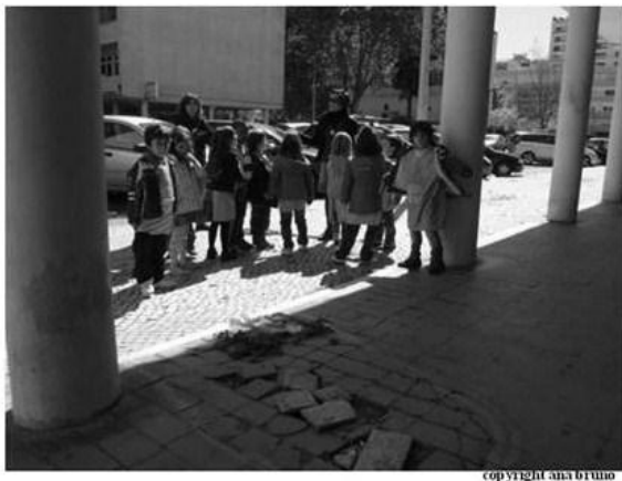
4. Observing a damaged pavement marked with graffiti ink
