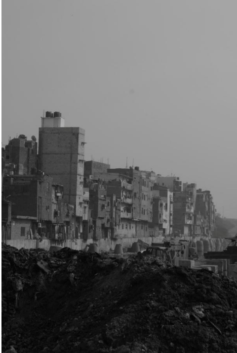
Delhi: work of infrastructural renewal. Image by Claudia Roselli.
