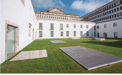
Figure 9. Interior patio and its lawn space with Department of Physics and University Archive in background.
