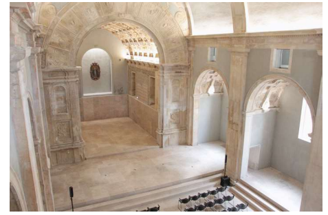
Figure 8. Interior of the Church of the Holy Trinity after restoration work
