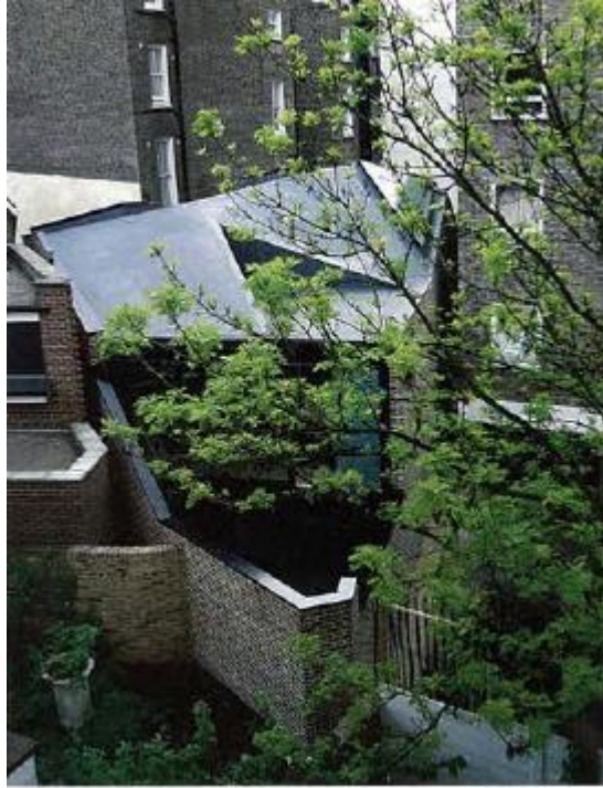
Fig. 26- Brick House vista exterior
