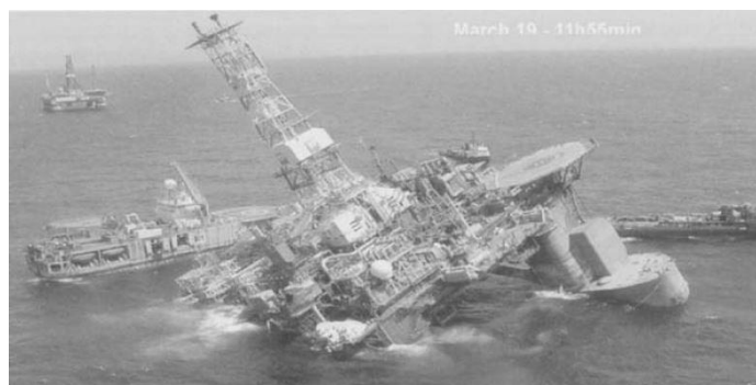
Figure 2.7 – Accident of P-36 converted semi-submersible after flooding in one column (Barusco, 2002).
