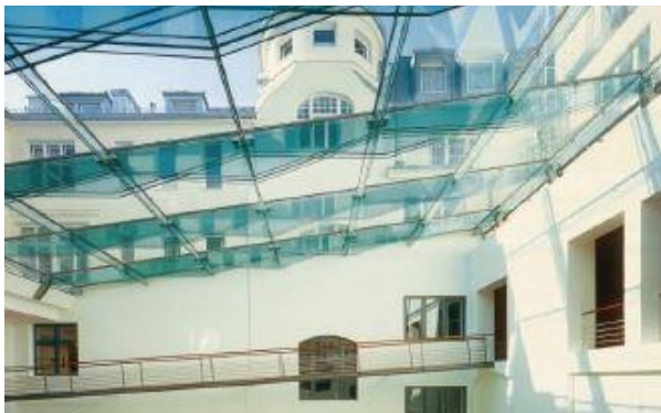
a) Structural glass applied in beams – Industrie Handelskammer, Munich, Germany [Image 5]
