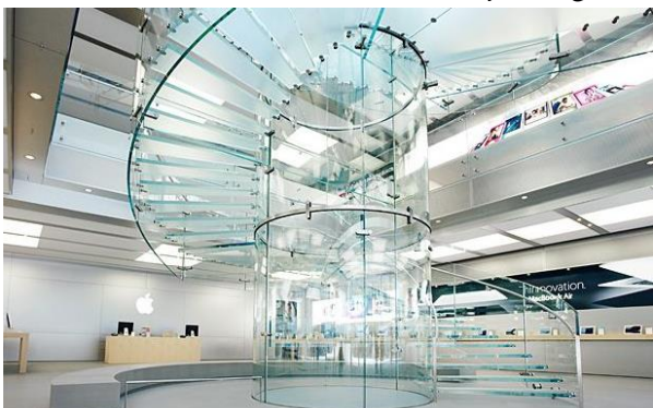
c) Structural glass applied in stairs – Apple store in 5 th Avenue, New York, USA [Image 7]
