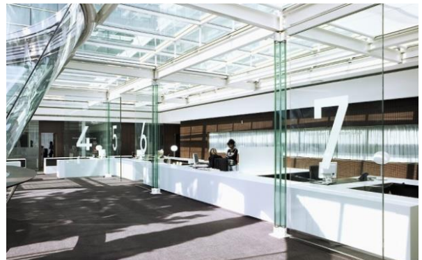
b) Structural glass applied in columns – St. Germain-en-Laye, France [Image 6]
