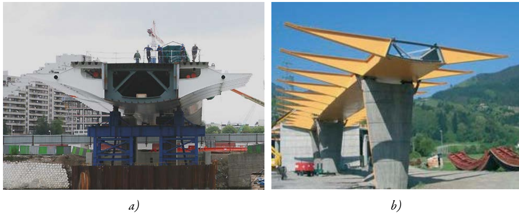
Figure 1.4: Curved cross-section of: a) Renault bridge (Boulogne-Billancourt) [11]; and b) bridge over the river Deba in Guipúzcoa [12]
