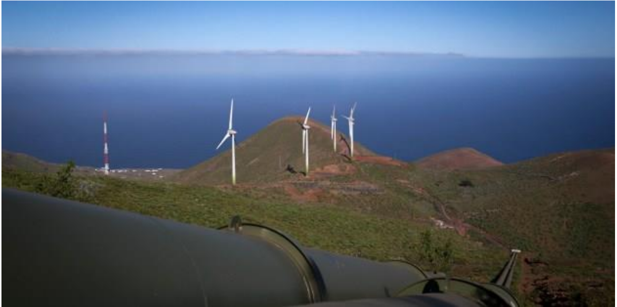
Fig. 14 – View of El Hierro’s pumped hydroelectric storage system, wind turbines and pipelines Source: LEW, 2014.
