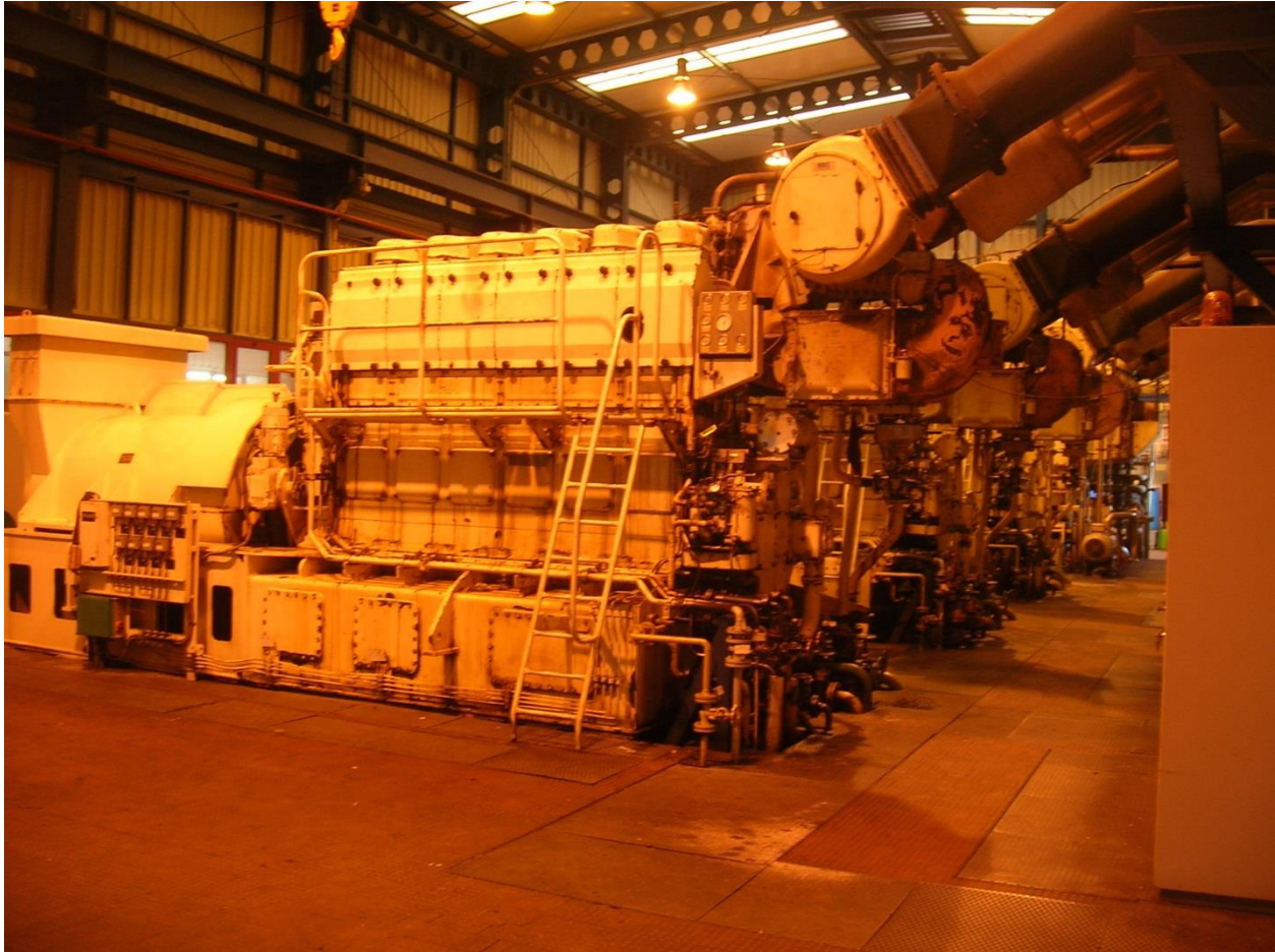
Fig. 24 – Diesel motors of the EDA central thermoelectric power plant in Sao Roque, Pico Source: Author of this article, 2017.
