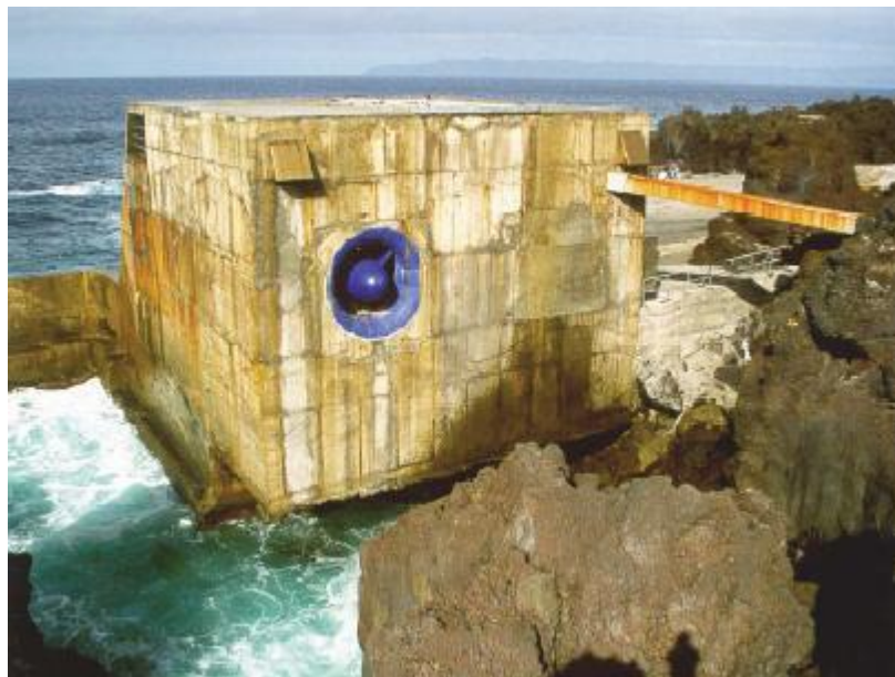
Fig. 27 – Pico's Oscillating Water Column wave energy plant in the village of Cachorro Source: RICO, 2009.
