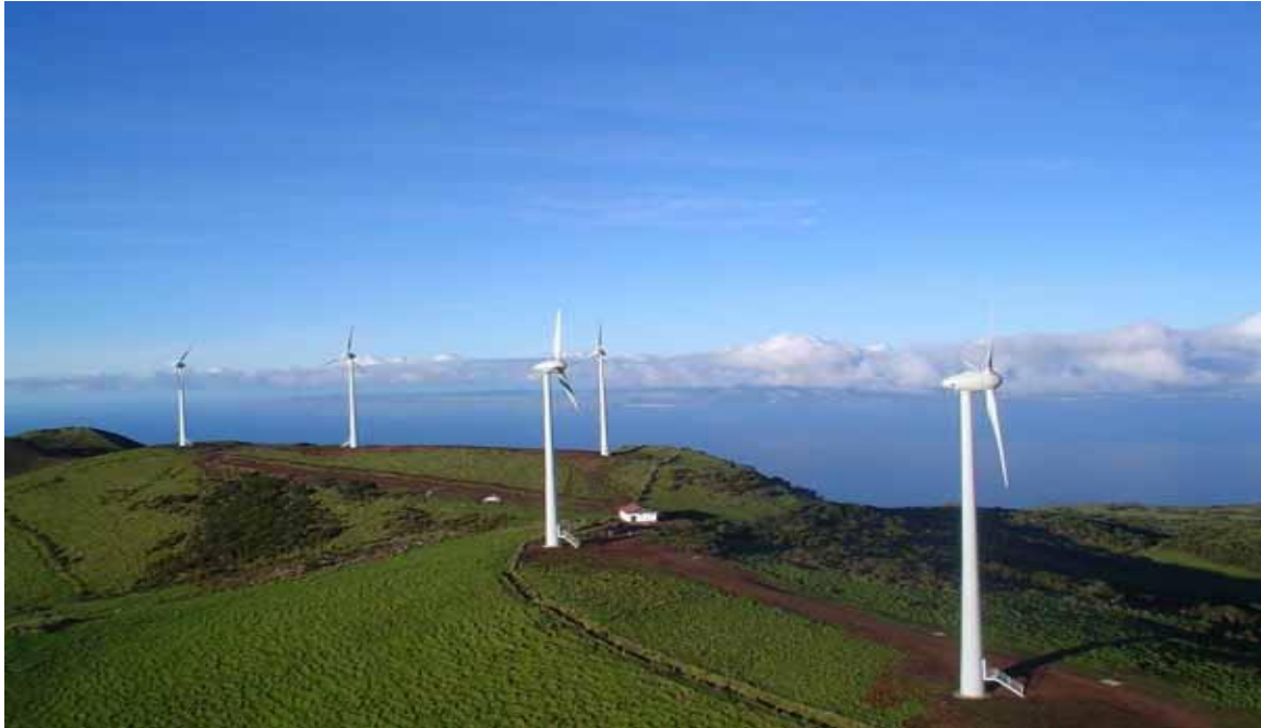
Fig. 25 - 5 of the 6 Enercon E-30/300 wind turbines that make up the Terras do Canto Wind Park on Pico Source: ENERGIASRENOVAVEIS, 2017.
