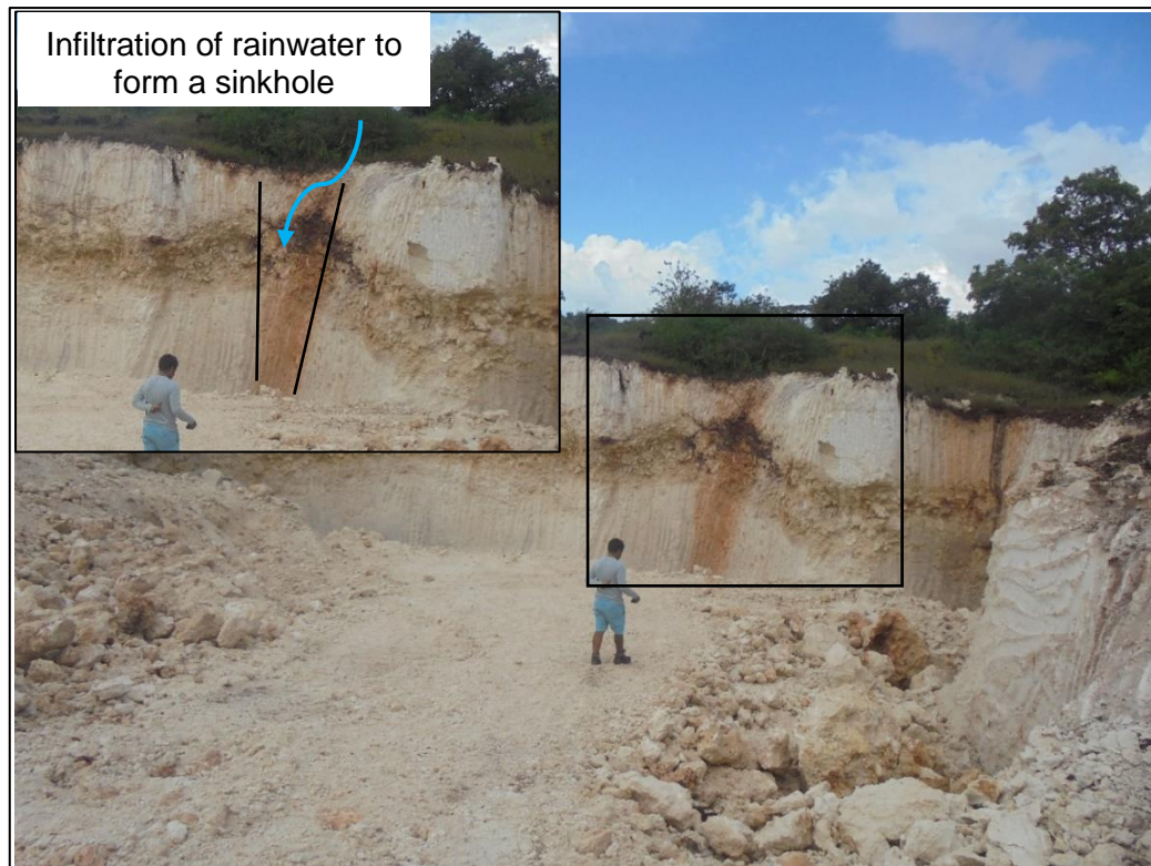
Figure 3. 12 Excavation Coral-reef of Baucau formation in the north plateau. Infiltration of rainwater dissolve through the crack of coral-reef limestone and will continue formed a sinkhole
