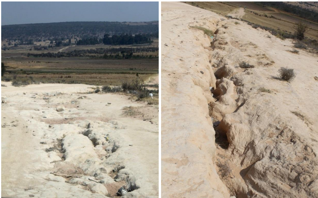
Figure 3.5 – Roads in Neves Dam area
