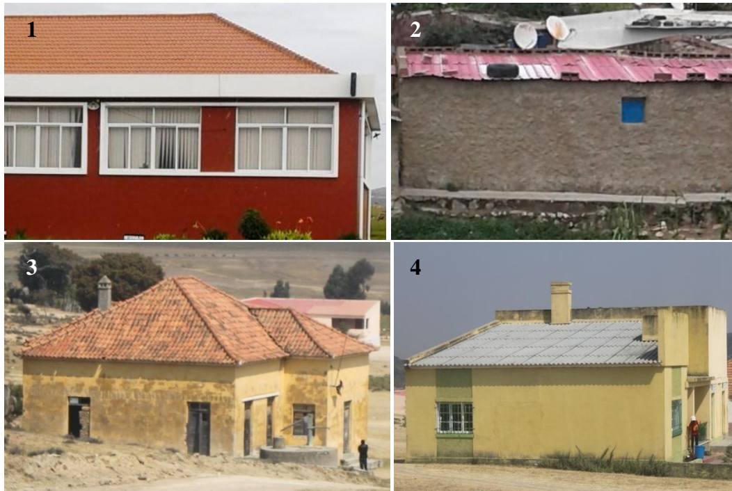
Figure 3.4.12 – Kinds of roofing: (1) new clay tiles, (2) pink coated metal sheeting, (3) old colonial clay tiles, and (4) asbestos roofing sheets
