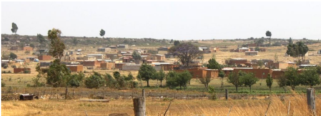
Figure 4.10 – Rural construction near Humpata
