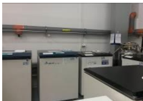
Fig 24 – Room with the freezers
