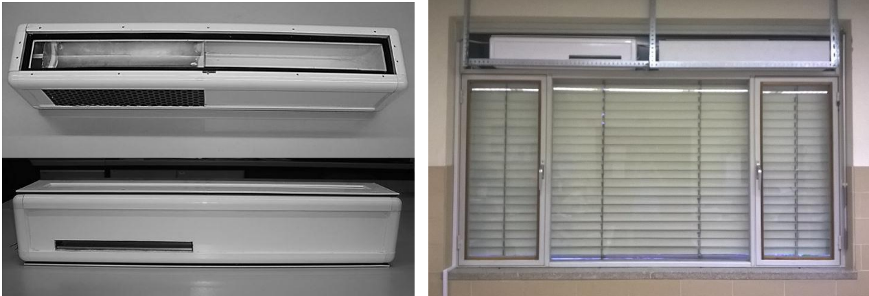
10 11 12 13 14 15 16 17 18 19 20 21 22 23 24 Figure 10 - Prototype of the mechanical ventilation subsystem of the Smart Window hybrid ventilation system. 25 26
