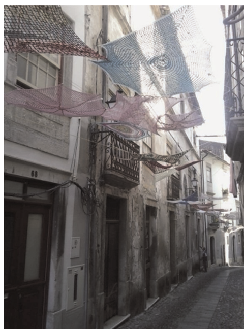
Fig. 1. “Casa das Talhas” (“House of cereals clay pots”).
