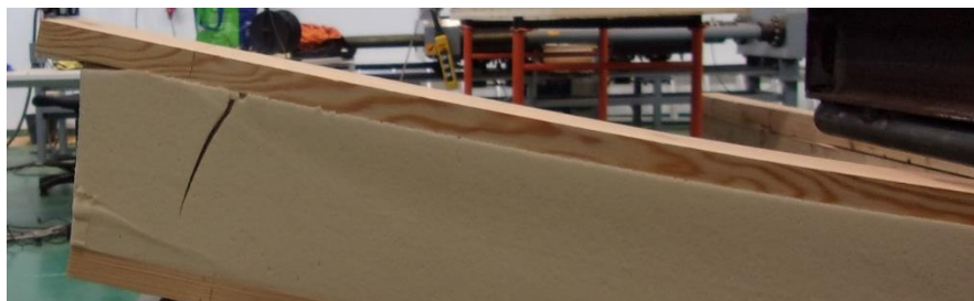
Figure 5-15 – Failure of SIP-20/120-B1.
