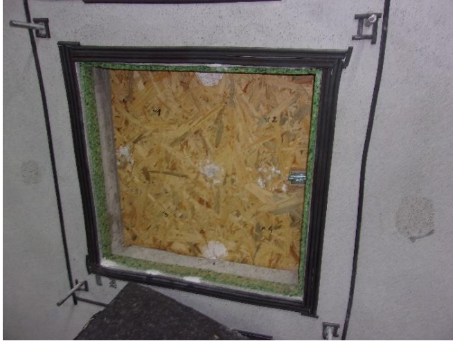
Figure 8-21 – OSB door at the inside of the chamber.
