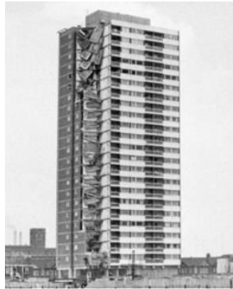
Figure 1-1: Ronan Point Tower partial collapse (Cook, 2018)
