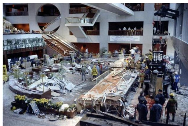
Figure 1-2 Hyatt Regency Hotel walkway collapse (MURPHY, 2014)
