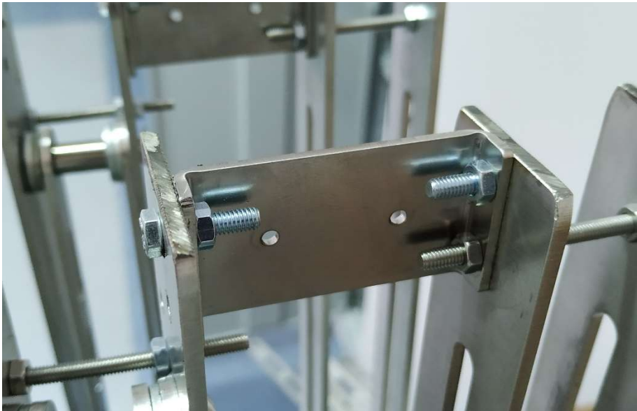
Figure 2.17. Pieces used to space bars.
