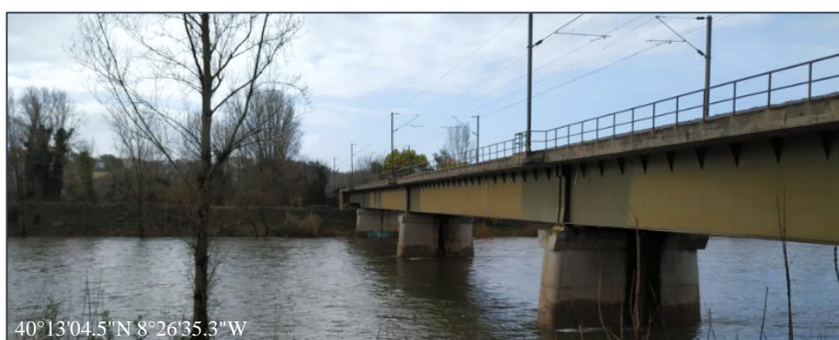
Figure 3.9 – Bridge over the Mondego River
