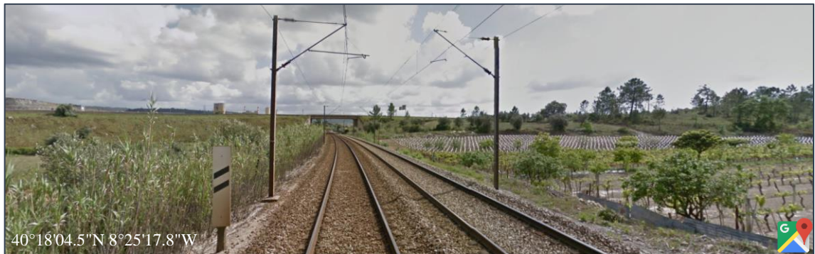
Figure 3.31 – Old signalling 5 km south of Pampilhosa (Google Maps)
