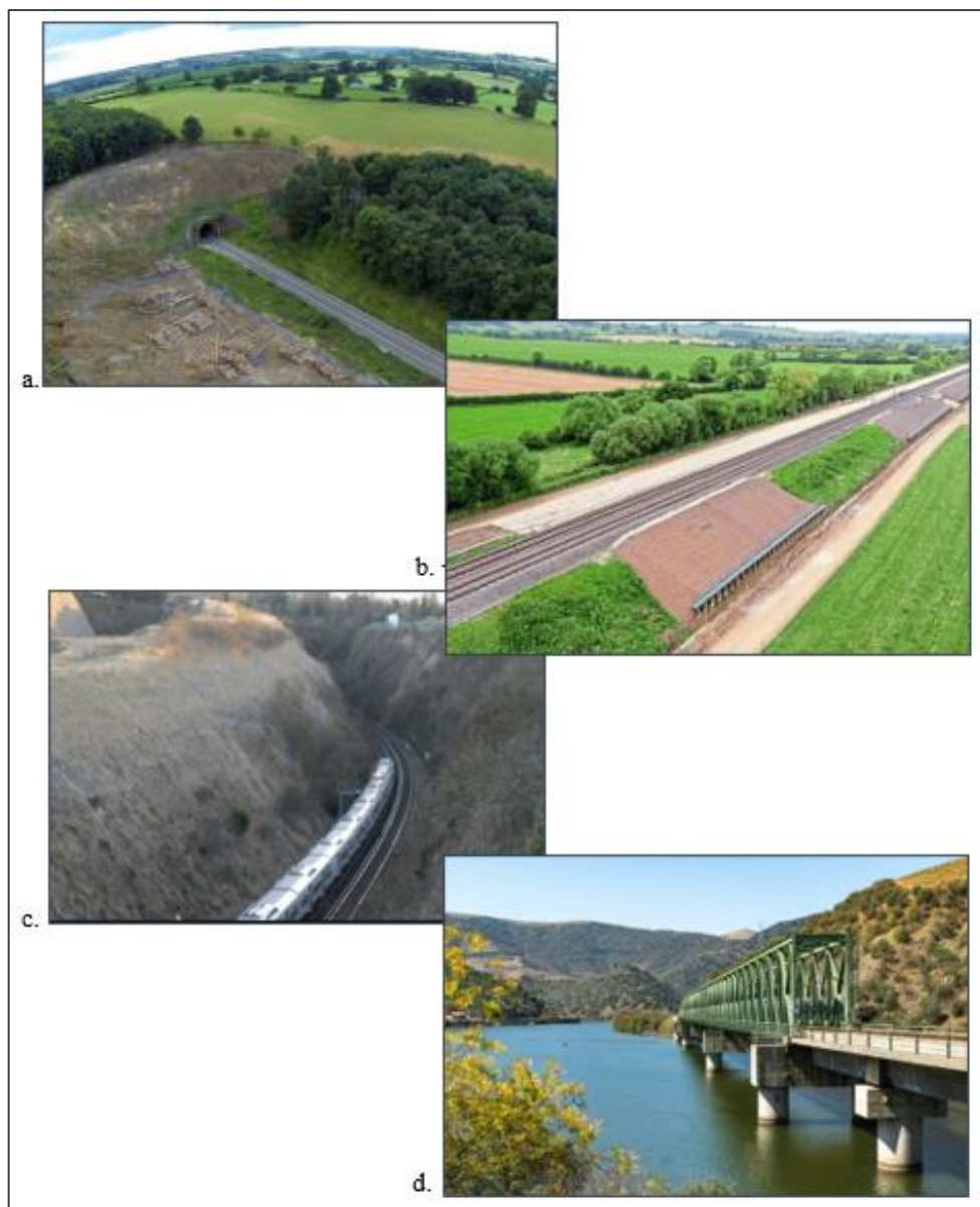
Figure 2.6 – Earth assets: a. Tunnel; b. Embankment; c. Cutting; d. Bridge (a. and c. Network Rail, 2020b; b. Keenan et al, 2019; d. Douro, 2020)
