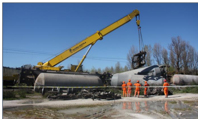
Figure 3.21 – Train derailment in Adémia, 2017 (Trainspotter, 2019)
