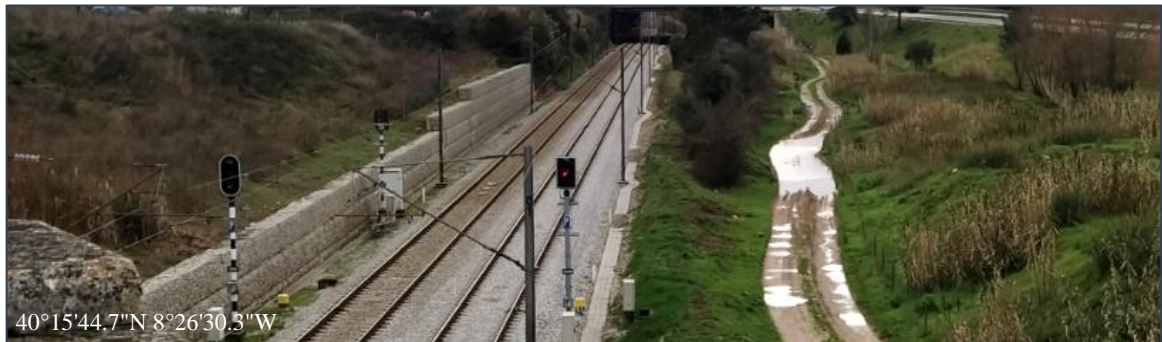
Figure 3.34 – Gabion retaining wall in Vilela
