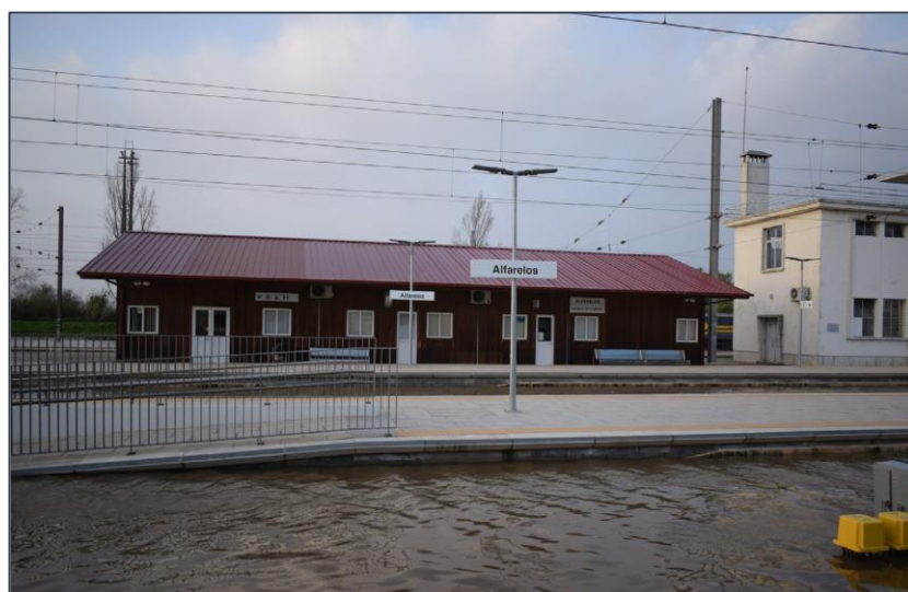
Figure 3.18 – Alfarelos train station flooded, 2019 (Cunha, 2020)
