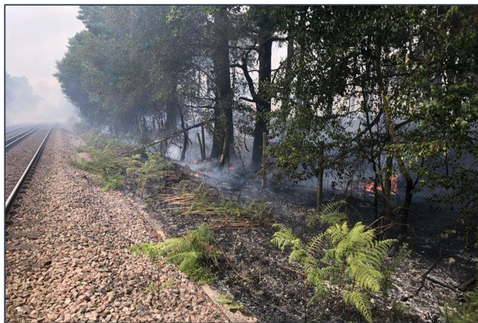
Figure 2.14 – Wildfire next to the railway track, UK (Network Rail, 2020b)
