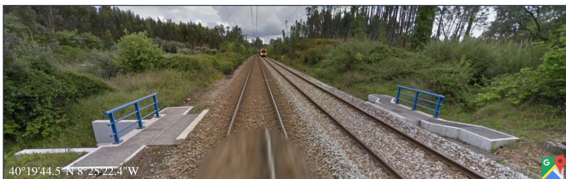
Figure 3.36 – Drainage system near Pampilhosa (Google Maps)
