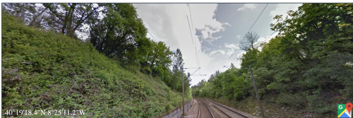
Figure 3.26 – Topped trees compared with vertical catenary poles (Google Maps)
