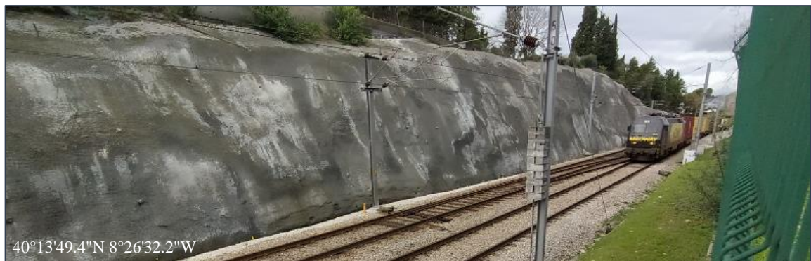
Figure 3.35 – Horizontal drains in Loreto
