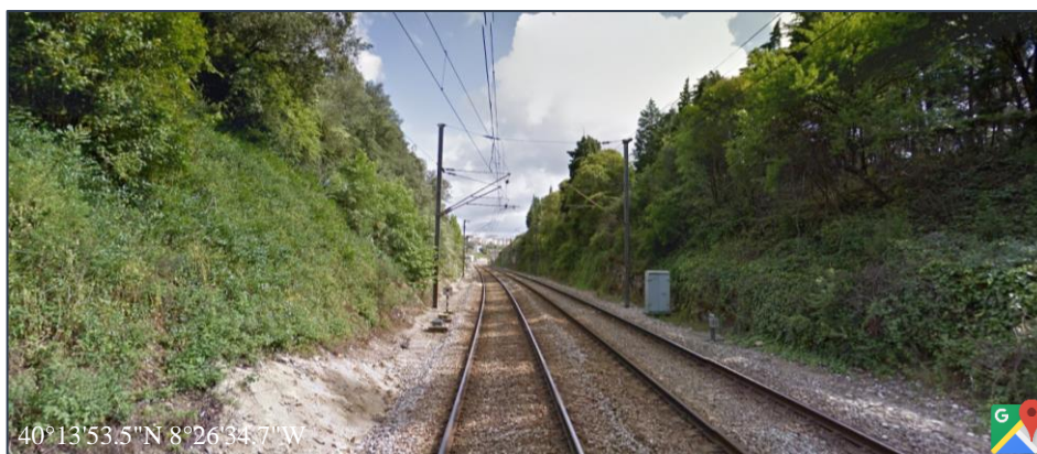
Figure 3.7 – Cutting to the north of Coimbra (Google Maps)
