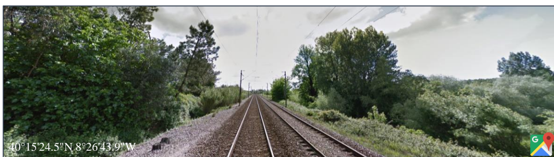
Figure 3.37 – Proper maintenance of vegetation near the railway (Google Maps)
