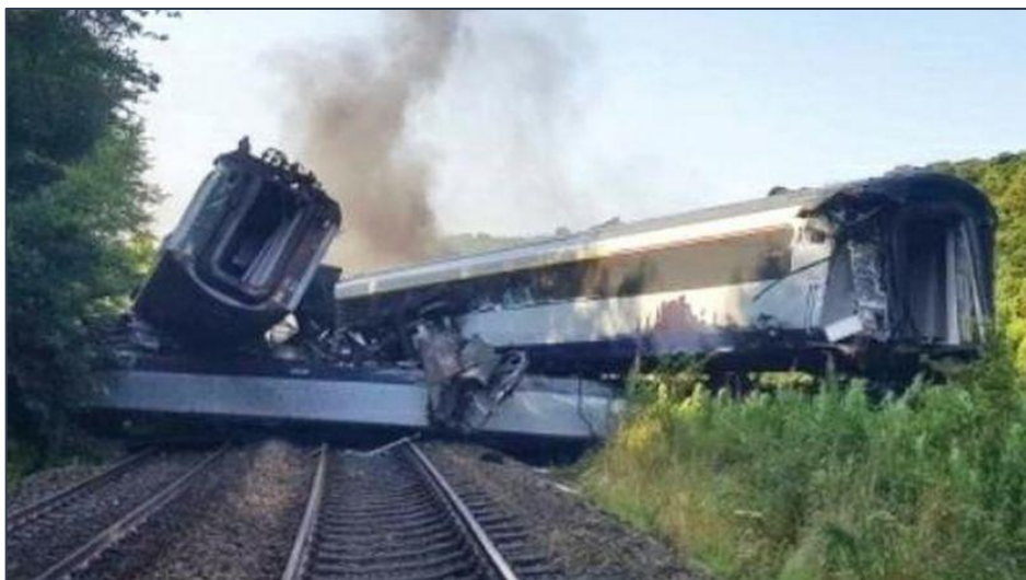
Figure 2.9 – Train derailment caused by a landslide, UK (Topham, 2020)
