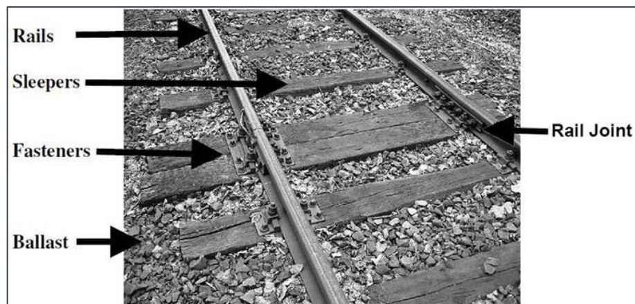
Figure 2.4 – Railway track (AGICO Group, 2020)
