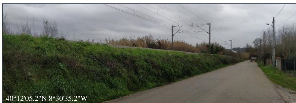
Figure 3.8 – Embankment to the west of Coimbra
