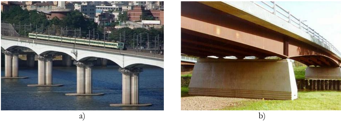
Fig. 1.1: Bridge decks with variable depth: a) Dangsang Bridge (South Korea, 1999) [1]; and b) Westgate Bridge (the UK, 1974) [2]
