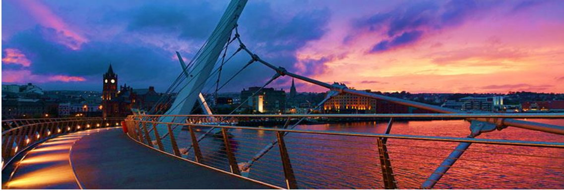
Figure 10 Peace Bridge in Derry, Ireland.
