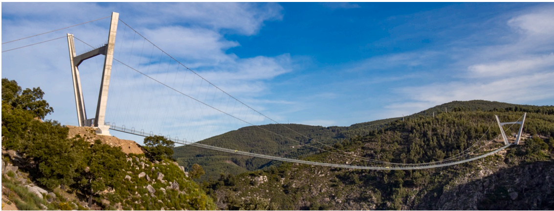
Fig. 1. View of the 516 Arouca footbridge (Portugal).
