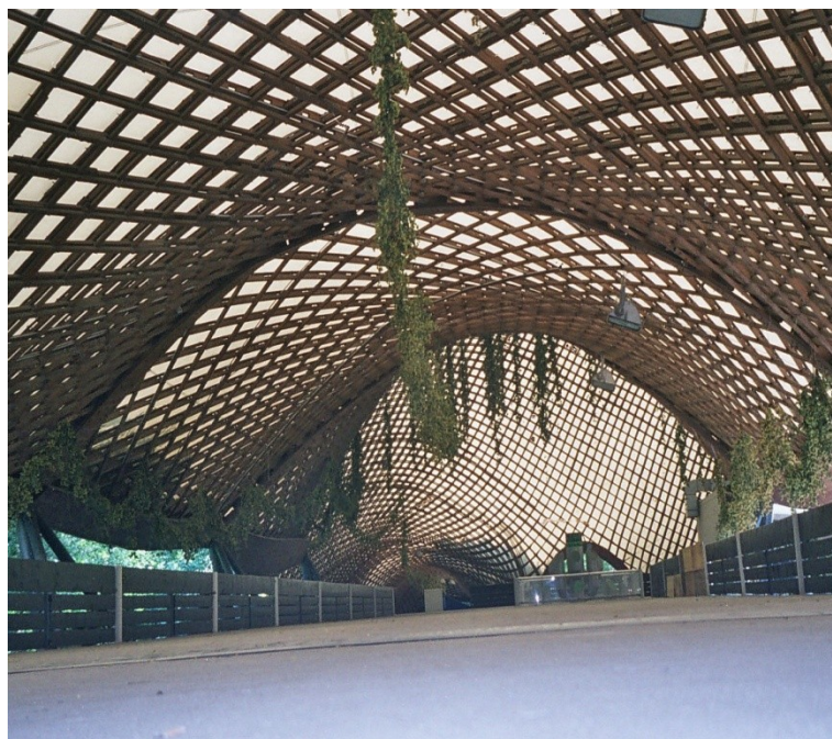
Figura 2.2 – Vista interior do Multihalle (Annular, 2002)
