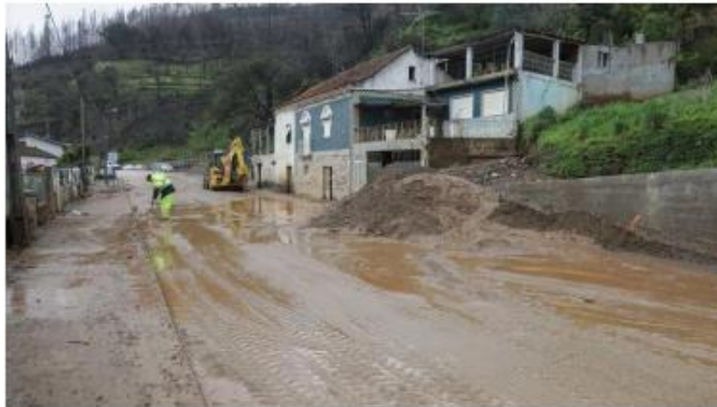
Figure 3: Accumulation of deposited material on Estrada da Beira (2018); Source: TSF (2023)
