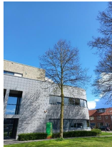
Figure 29: Building B, photo by author
